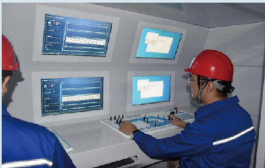
Monitoring operation center (inside)
